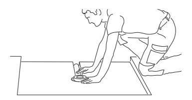
2) The base element is trimmed from the edge towards the area of the DN 50 discharge pipe with the help of a saw.
