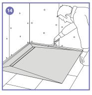
14. Build up the surrounding floor area with Jackoboard Construction Board (10mm) to bring it level with the shower base and then seal and tape all joints with an appropriate sealing system (such as the Jackoboard sealing Set) for example.
